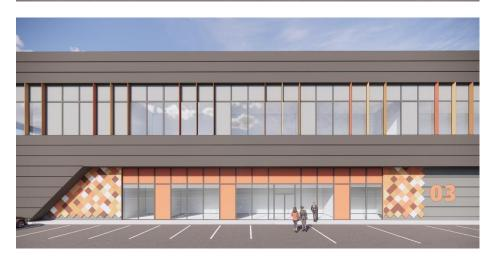
Given that the area of the first floor of the admin block is larger than the ground floor, the façade steps out to the front and over the loading bay to give a cantilevered appearance and to frame the entrance. The Admin Block is clad horizontally fixed, composite flat metal panels with mineral wool core, powder coated to a dark grey colour at first floor and light grey at ground floor.
