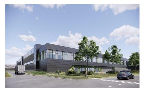
The Data Hall is clad with horizontally fixed, composite flat metal panels with mineral wool core, powder coated to a range of grey colours. The image below shows the long façade and the use of a variation of colours to break up the façade. There is a gradient of colours from the base of the long façade getting lighter towards the parapet. Large louvered sections sit within the façade to provide ventilation to the AHUs internally.
